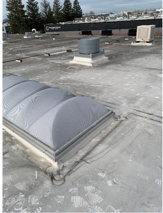
Single Ply Roofing
